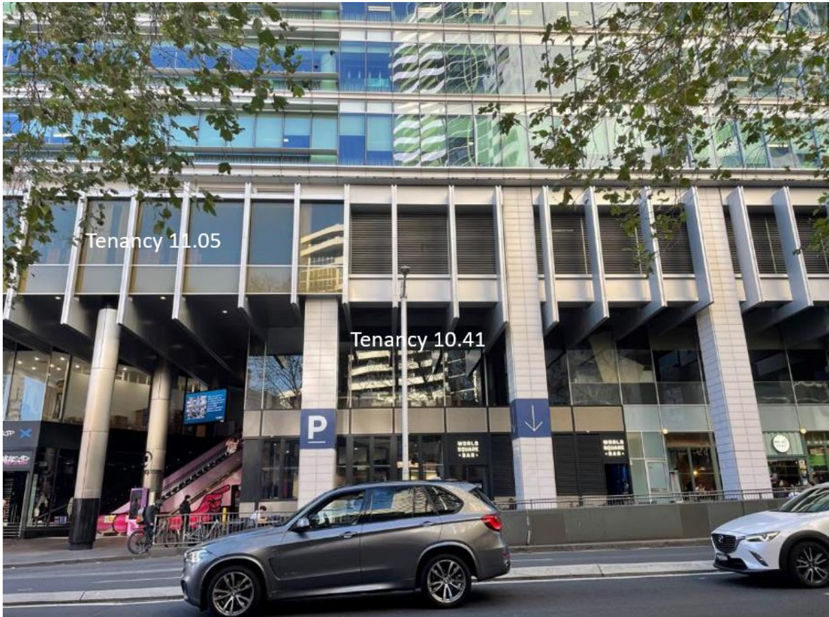
Figure 5: Site viewed from Goulburn Street
